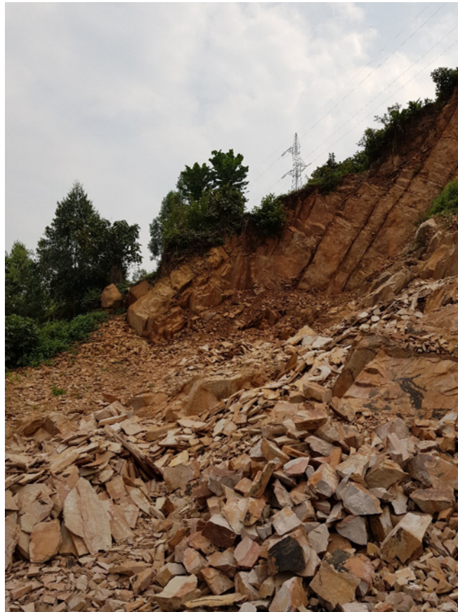
Picture 4: Quarry with adjacent electricity tower
