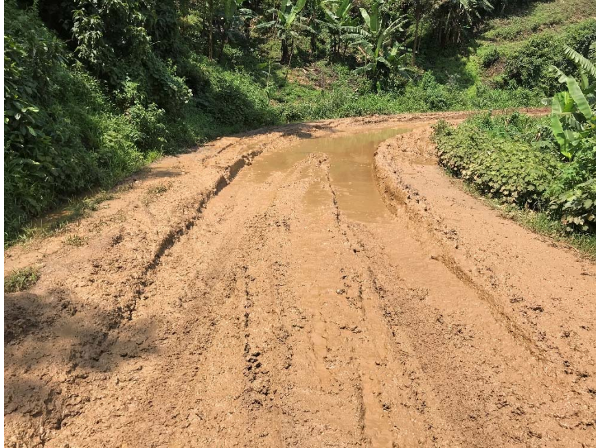
Picture 7: Area of poor road condition along RN2
