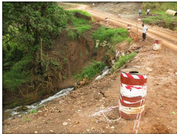
Figure 2.7: Inappropriate hazard demarcation
