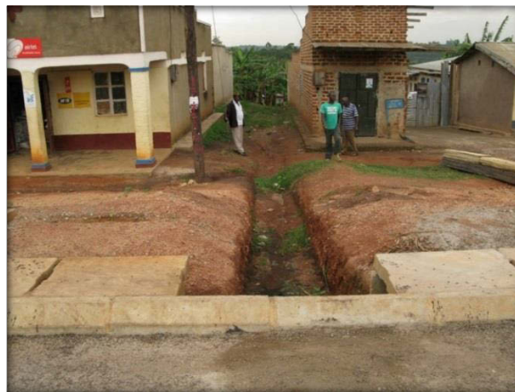
Figure 2.4: Inappropriate location for discharge from covered roadside drain
