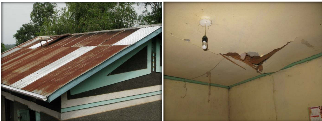
Figure 2.6: Roof repair (left) and unrepaired ceiling (right), both damaged by flying rock from the Busima-Bigodi quarry
