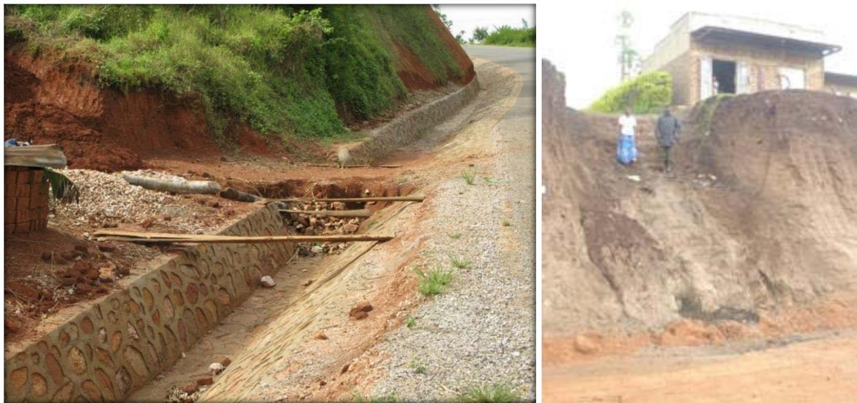
Figure 2.2: Informal access to road across deep, stone-faced drain (left) and dangerous access to occupied properties (right) 69
