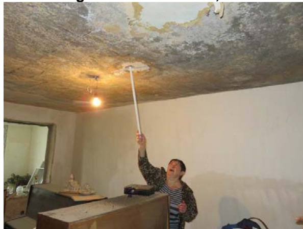
Figure 5: Ceiling in Flat 30 under the roof. Heavily decomposed, visible deflection, insufficient concrete coverage of reinforcement, removable with a broomstick.
