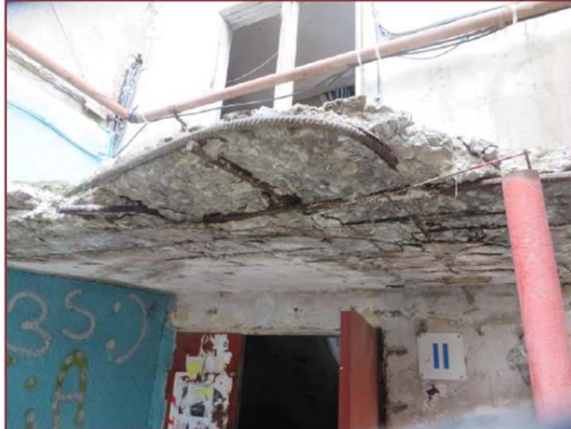
Figure 4: Porch at the entry of staircase number 2. Small parts of concrete are falling down continuously. The whole substructure is prone to break down. The steel bars of the reinforcement are visible without concrete coverage. Deformations due to decomposition of the concrete element are visible.
