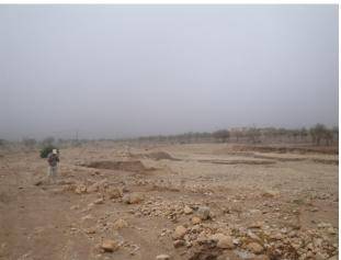
In conclusion, the complaint is justified. As part of the rehabilitation of building materials extraction sites and during site cleanup, the Contractor must carry out corrective works, strengthen the dike, refill eroded banks and remove stones carried and deposited by floods on land immediately downstream from the dike.
