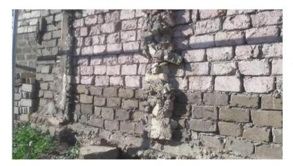
This wall used to be an "internal" wall but is now external and causes rain water seeping into the house.
