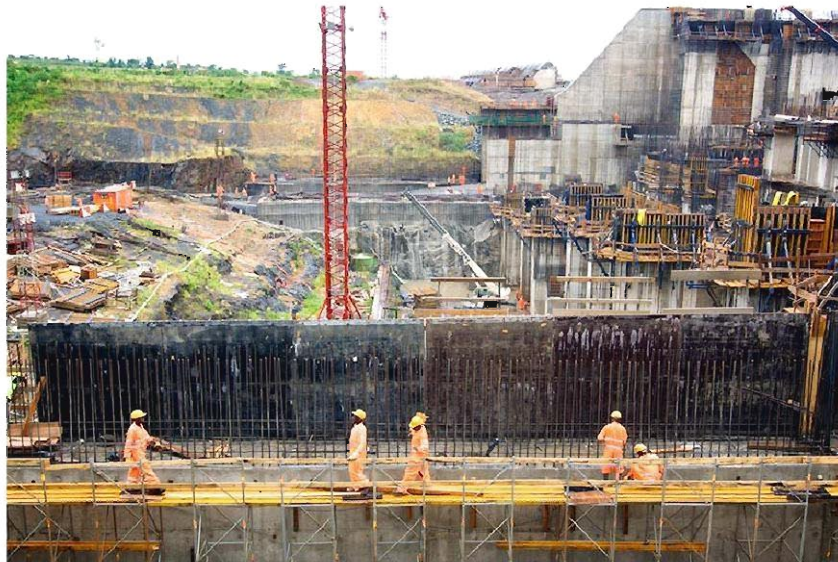
The Bujagali Hydroelectric project in progress
